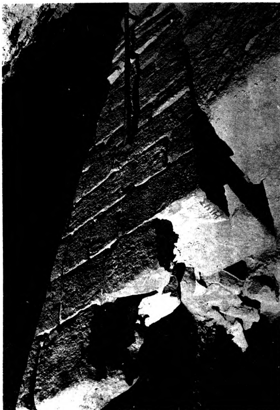
G. The outer peripheral wall.
